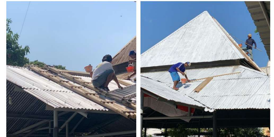
After cool roof paint application
