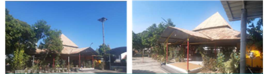
Before cool roof paint application
